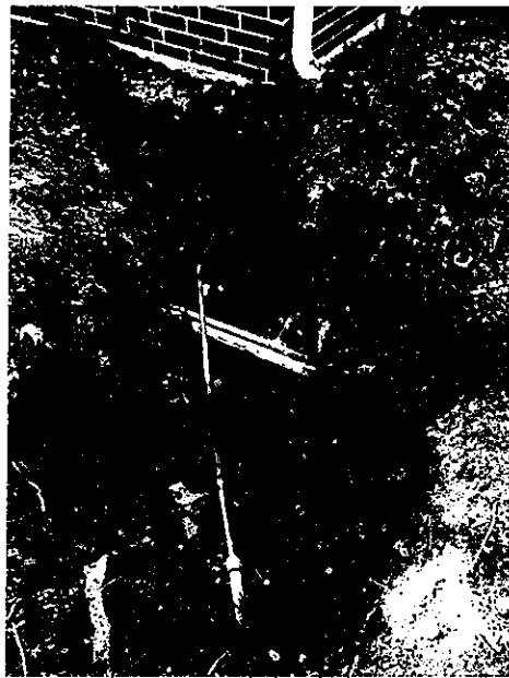
Repair of leak
