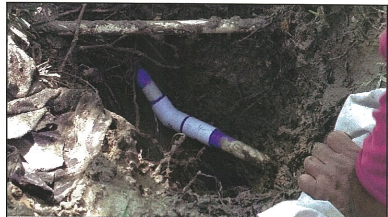
18 April 2018 – Repair made by Bettencourt Plumbing of 45 fitting as it goes under the driveway slab.
