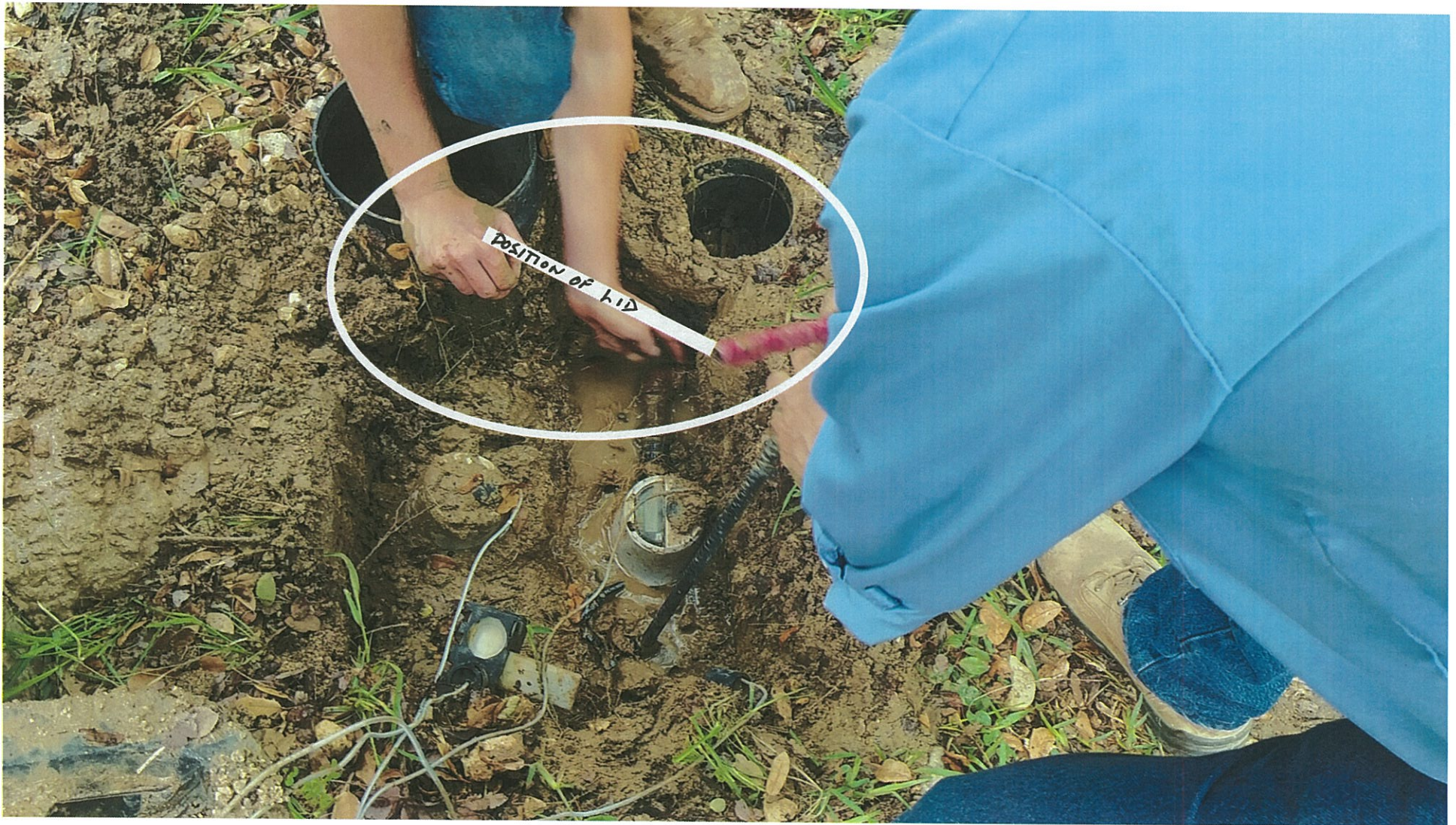
12 April 2018 – Approximate location of the iron utility cover discovered and removed by city water department personnel.
