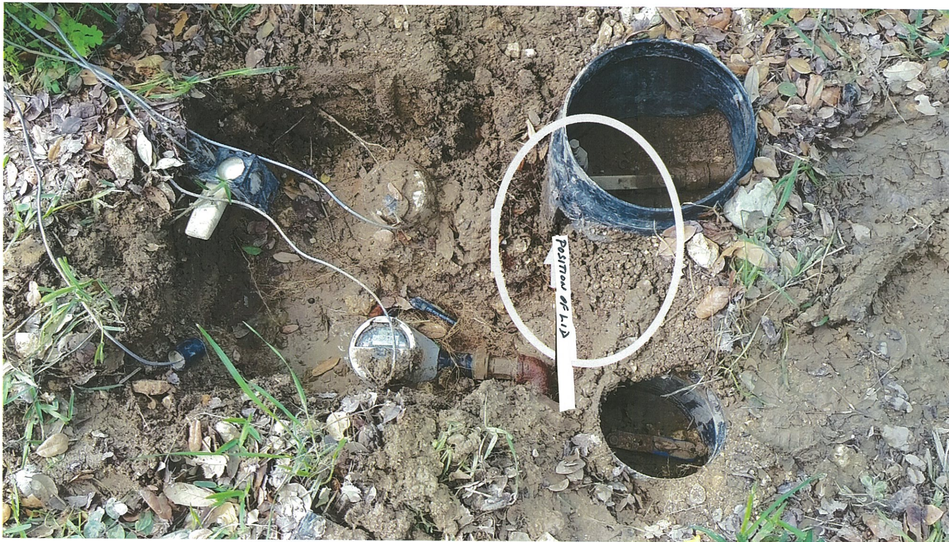
12 April 2018 – Clearer shot of the cutout on the larger valve box where the iron cover was inserted vertically.
