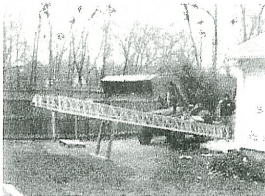
Here the tower is carefully moved with the help of a front end loader.
