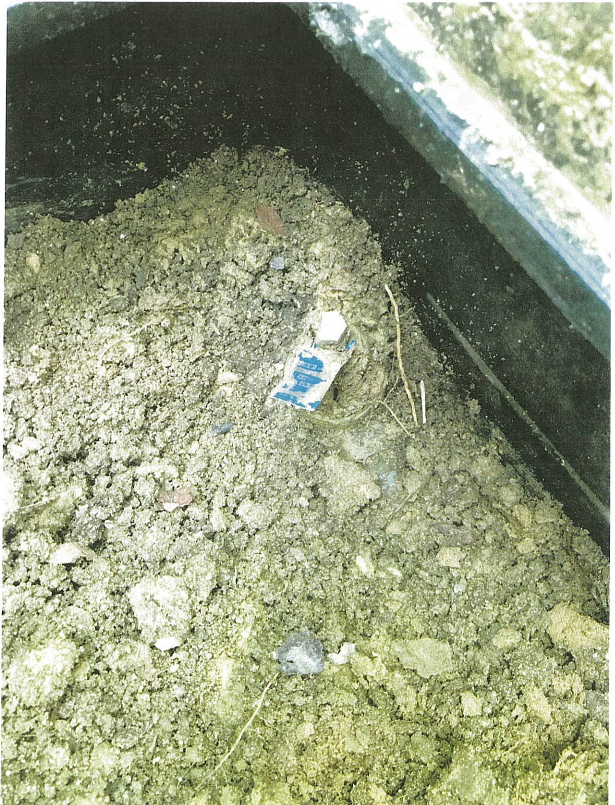
OLD PRESSURE REDUCING VALVE PHOTO #26
