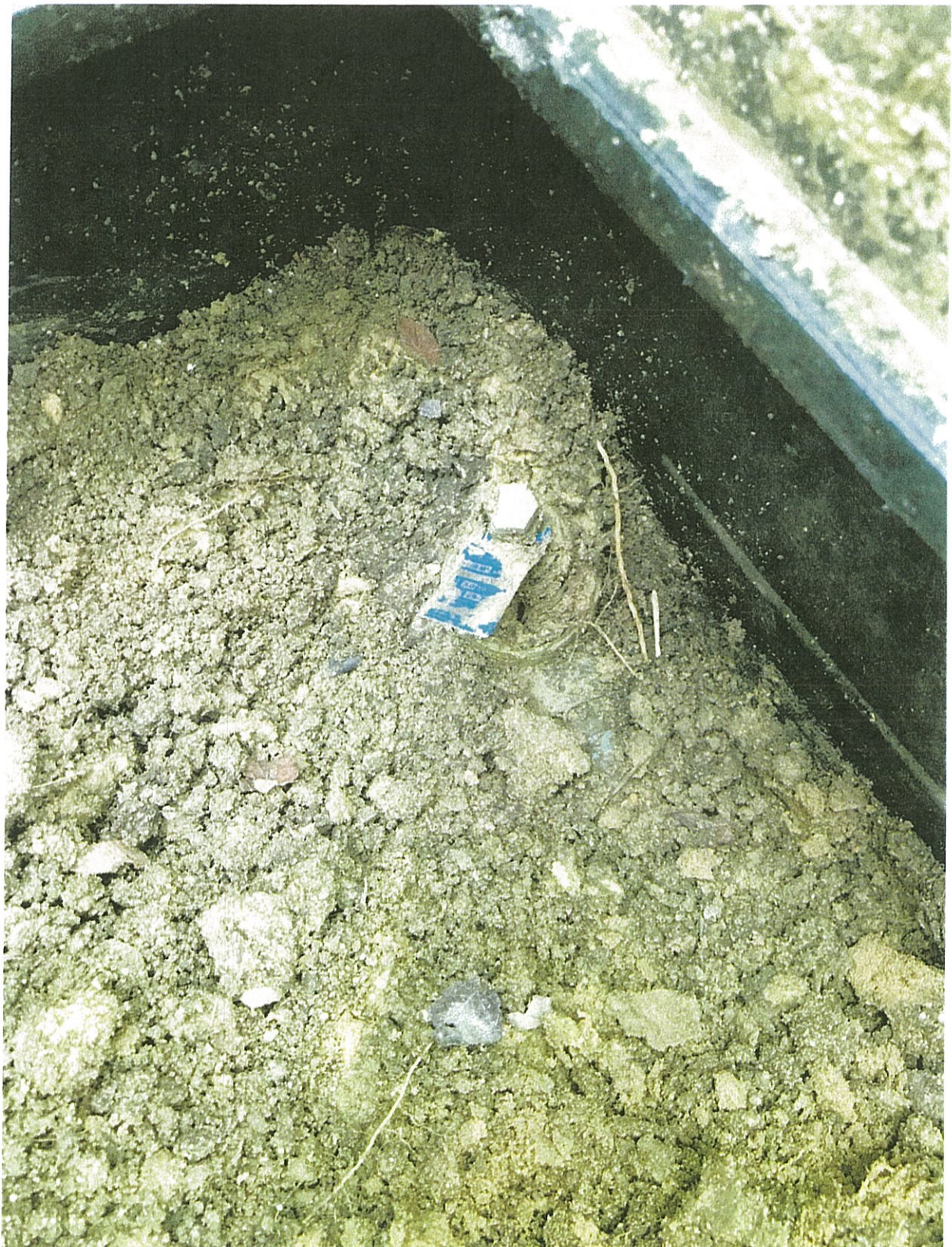
OLD PRESSURE REDUCING VALVE PHOTO #26
