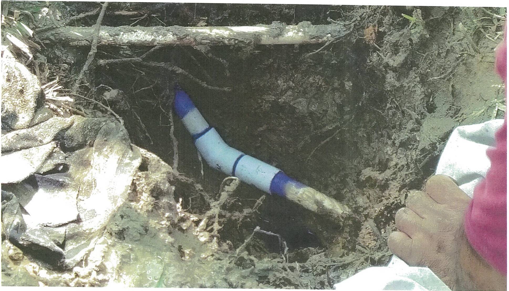
18 April 2018 – Repair made by Bettencourt Plumbing of 45 fitting as it goes under the driveway slab.
