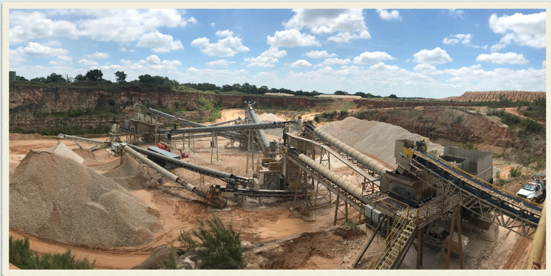
Dry Plant Crusher in enclosure
