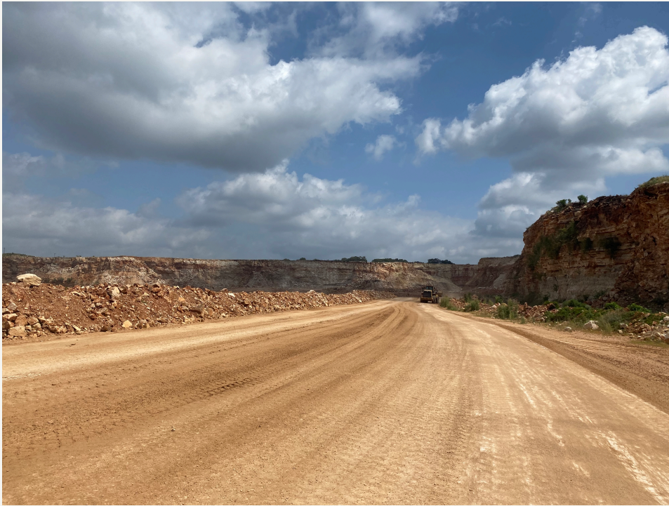
Wide haul roads saturated for dust suppression
