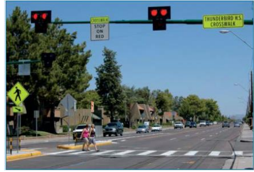
Pedestrian hybrid beacons offer clear guidance on when pedestrians may cross the street at a mid-block crosswalk and raise awareness to automobile traffic
