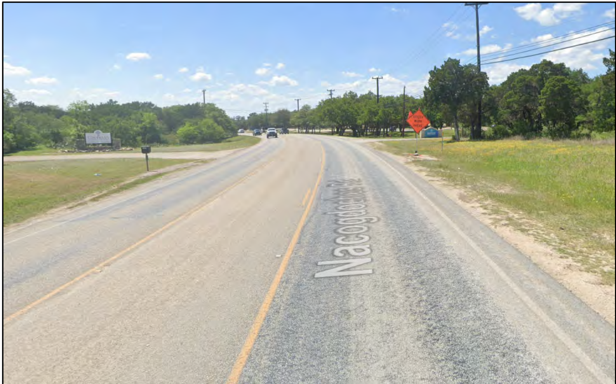
Figure 6. Nacogdoches Road (FM 2252) – Facing South from Hickory Bend
