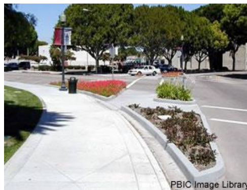
Reducing the curb radius, even in places without sidewalks, reduces the crossing distance for pedestrians and requires vehicles take the turn at slower speeds.
