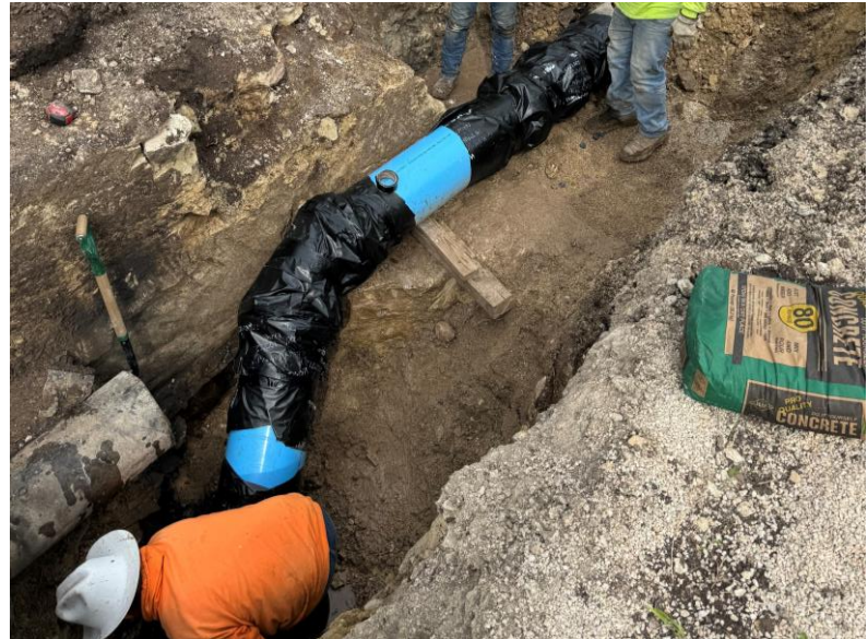
Alignment Adjustment east of Bat Cave Road
