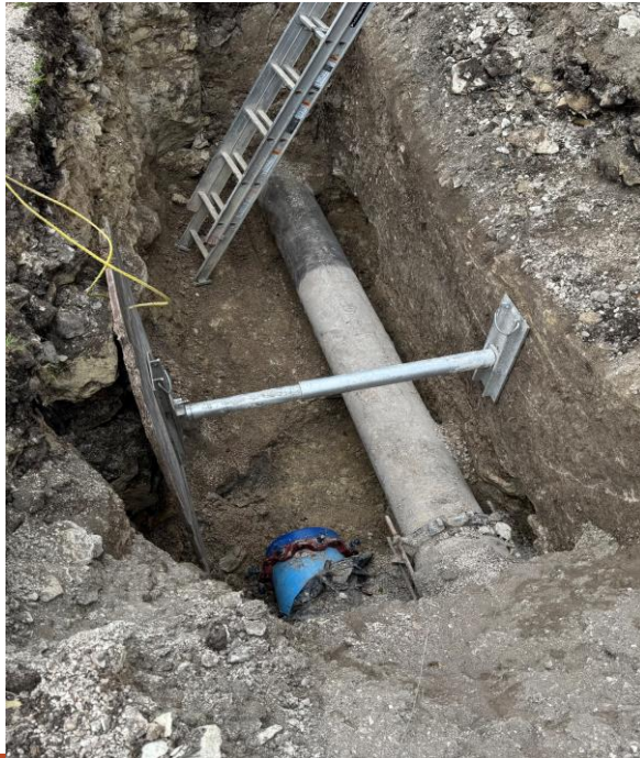
Alignment Adjustment east of Bat Cave Road
