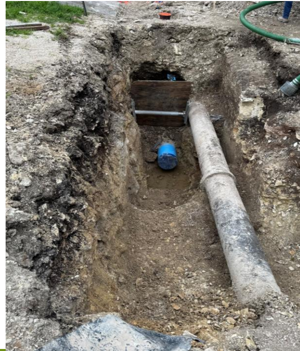
Alignment Adjustment east of Bat Cave Road
