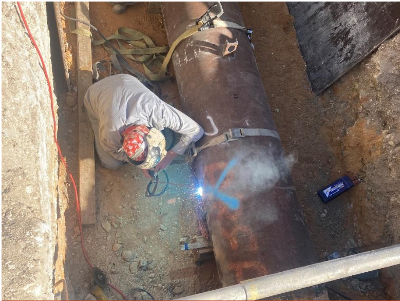
24" Steel Casing Extension at Bat Cave Road
