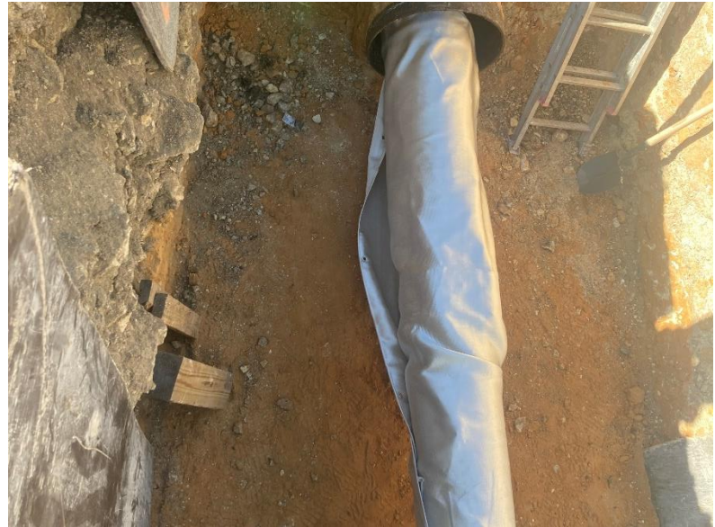
24" Steel Casing Extension at Bat Cave Road
