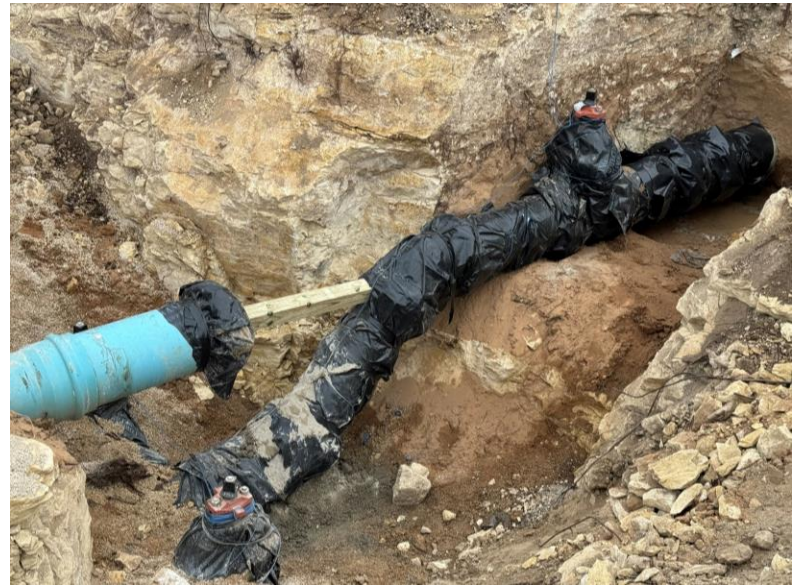
Tie-in connection point at Tonkawa Pass
