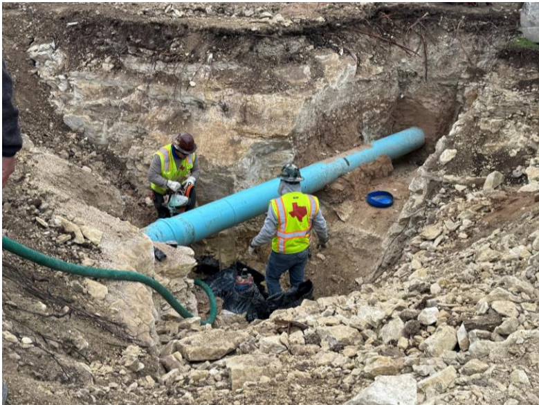
Tie-in connection point at Tonkawa Pass
