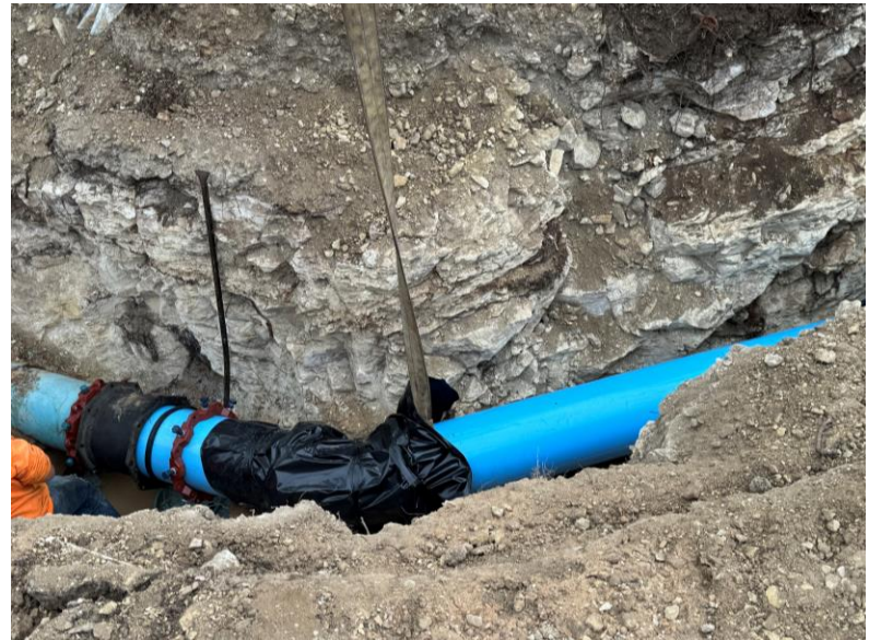
Tie-in connection point at Tonkawa Pass
