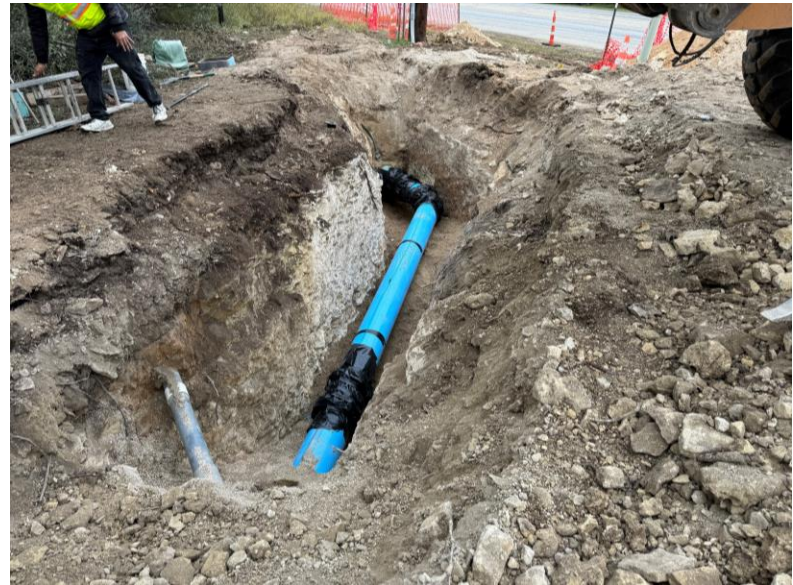
Tie-in connection point at Tonkawa Pass
