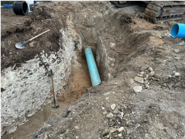
Tie-in connection point at Tonkawa Pass
