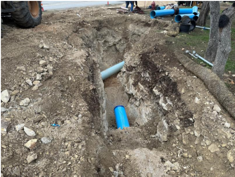
Tie-in connection point at Tonkawa Pass
