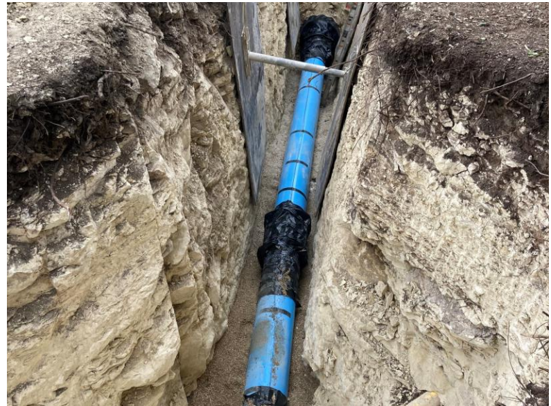
12-inch Main Installed at Tonkawa Pass Approximately STA. 182+39 to STA. 182+65
