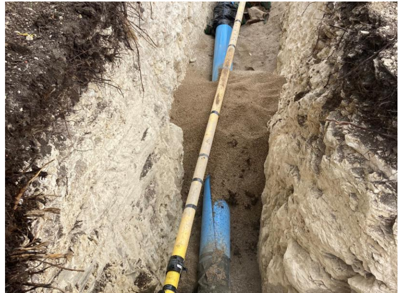
12-inch Main Installed at Tonkawa Pass Approximately STA. 182+65 to STA. 182+96
