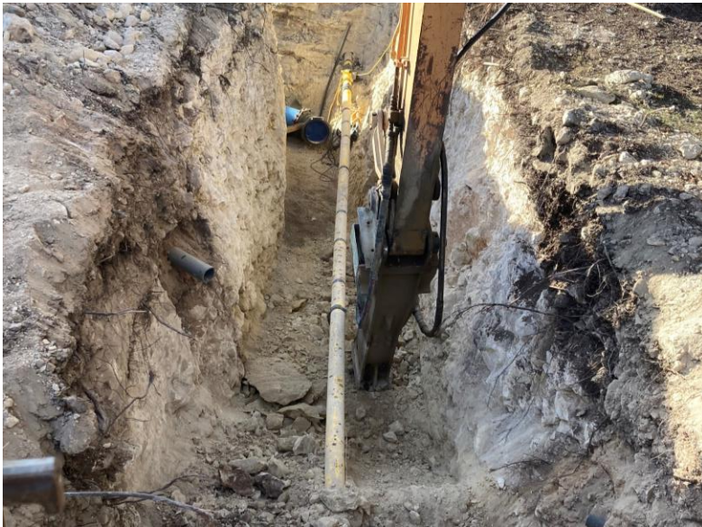
Trench Excavation for the 12-inch Main at Tonkawa Pass Approximately STA. 182+65 to STA. 182+96
