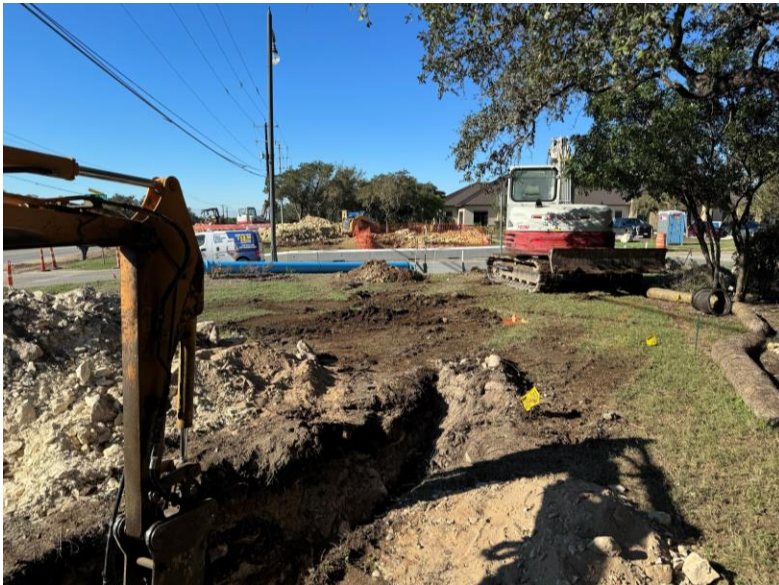
Trench Excavation for the 12-inch Main at Tonkawa Pass Approximately STA. 182+39 to STA. 182+65
