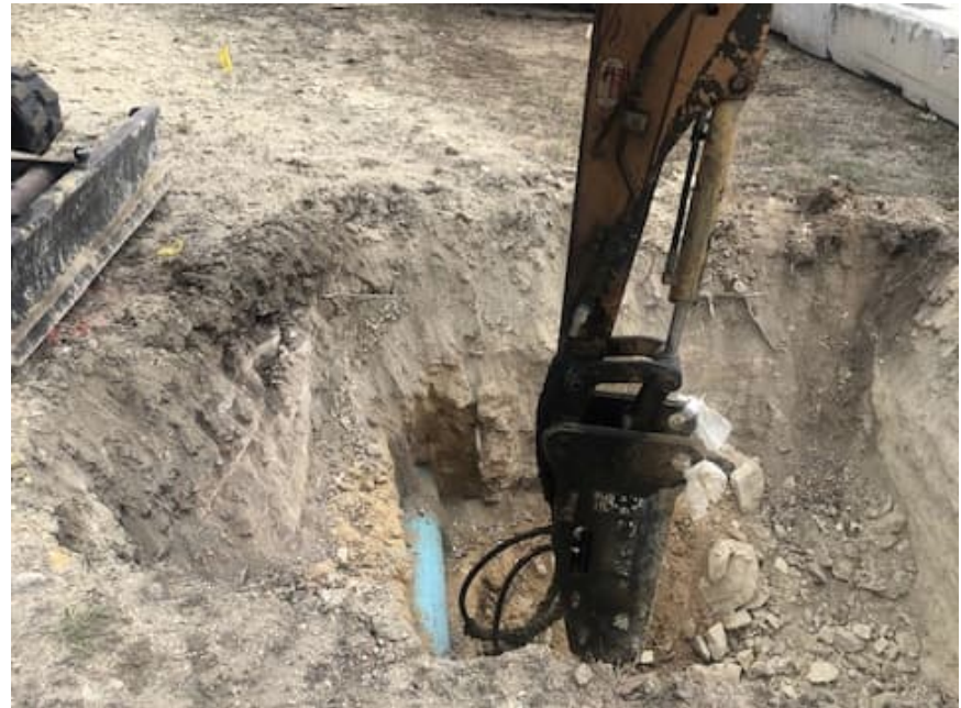
Preparing to Connect to Existing Main at Hickory Bend
