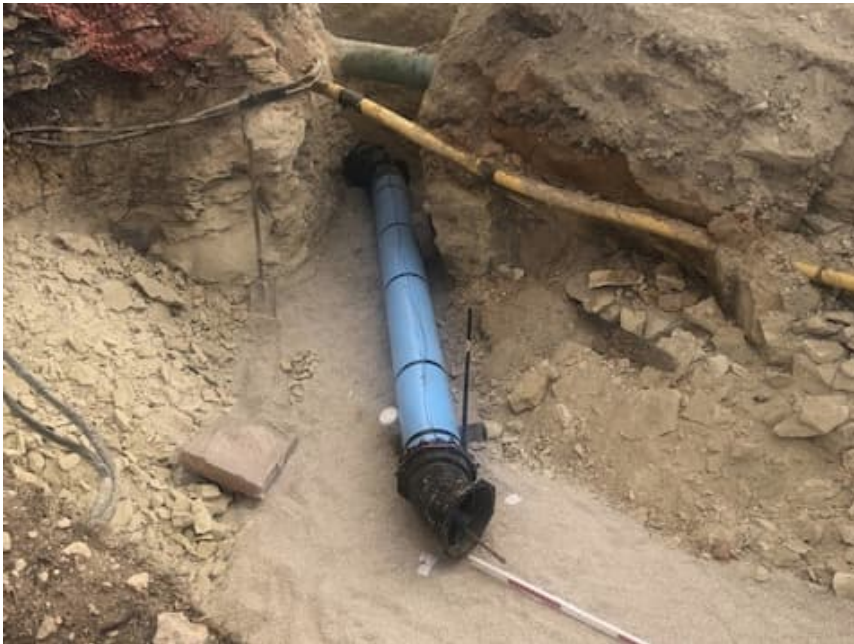
Approaching Casing Under Hickory Bend
