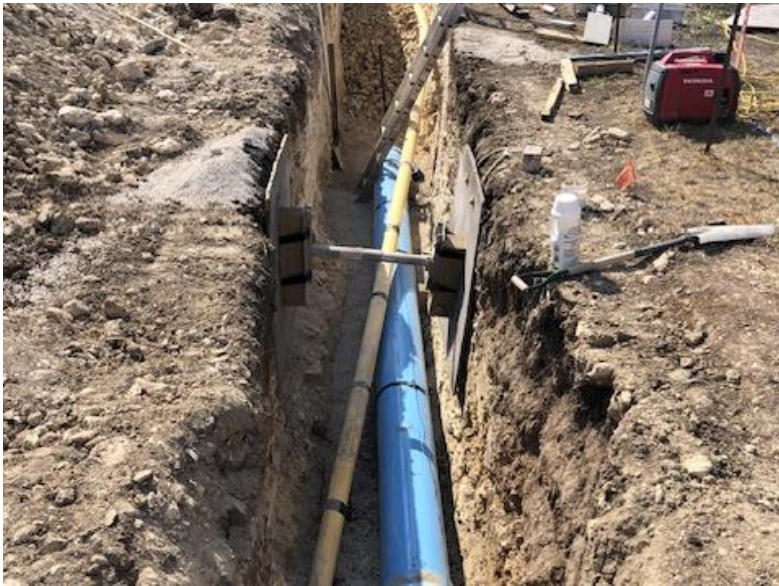
CenterPoint Gas Line Crossing Approximately STA. 233+00
