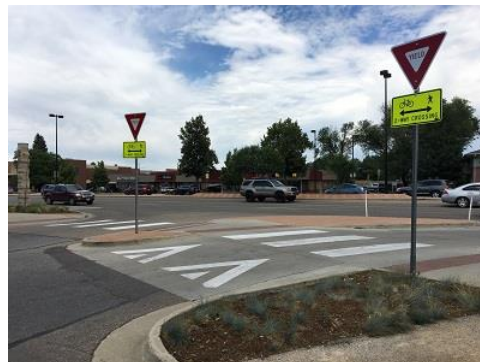
Raised crosswalks raise awareness and lower vehicular speeds on the approach to a crosswalk, particularly in areas like slip lanes.
