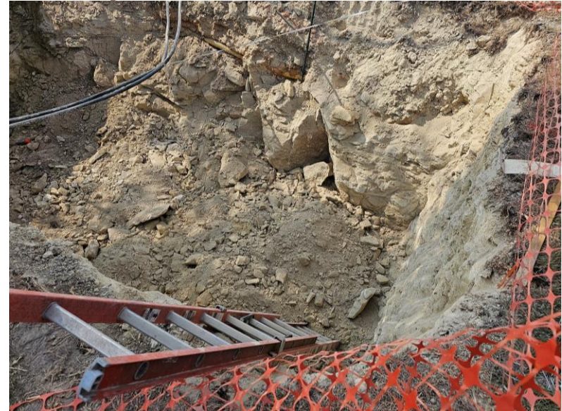
Hickory Bend Bore Pit Excavation
