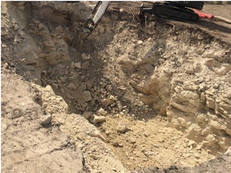
Tonkawa Pass Bore Pit Excavation Approximately STA. 181+91
