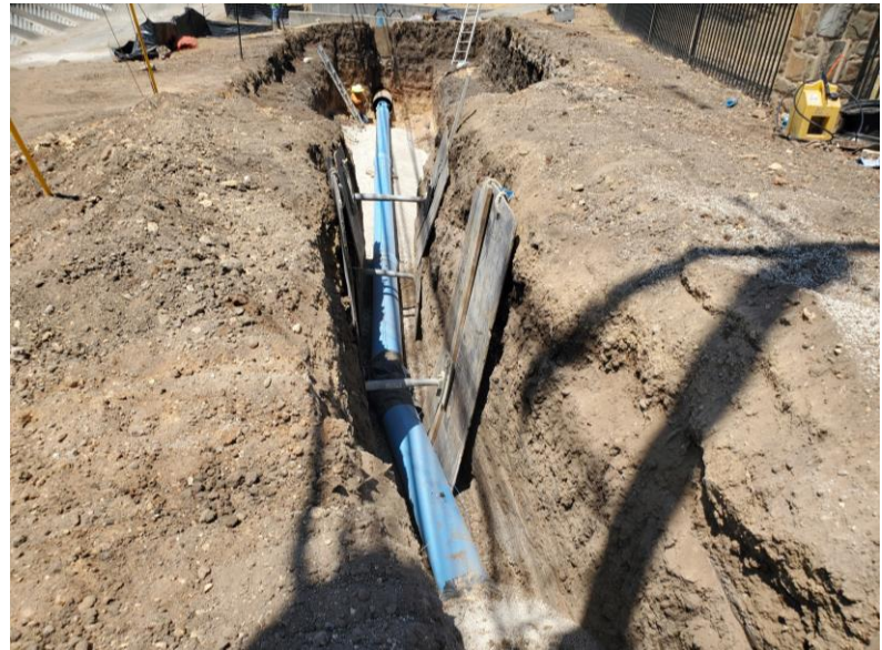
Water Line Approximately STA. 236+87 to STA. 237+44
