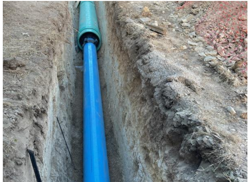
PVC Casing Under Driveway Approximately STA. 232+50
