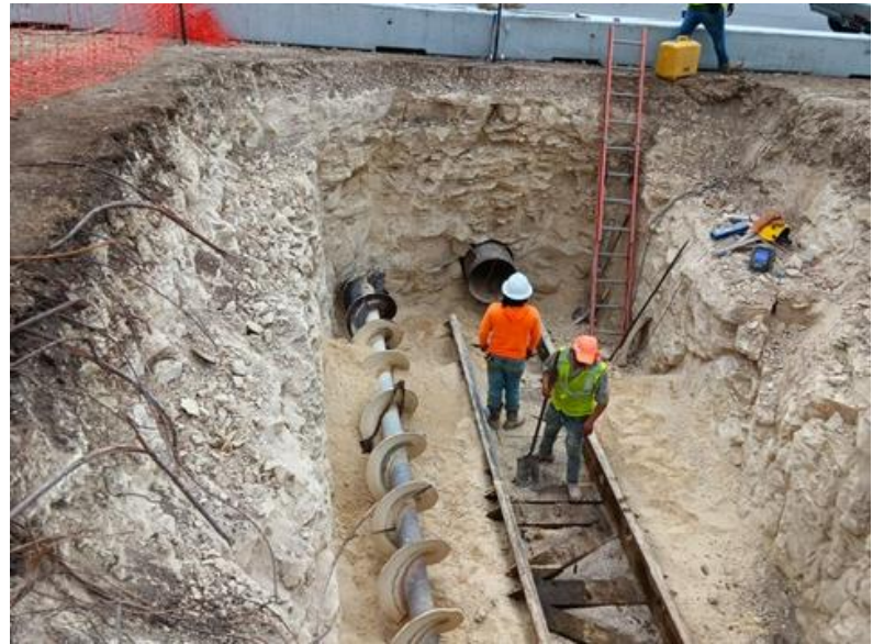
Bored 24-inch Steel Casing Under Tonkawa Pass Approximately STA. 181+91
