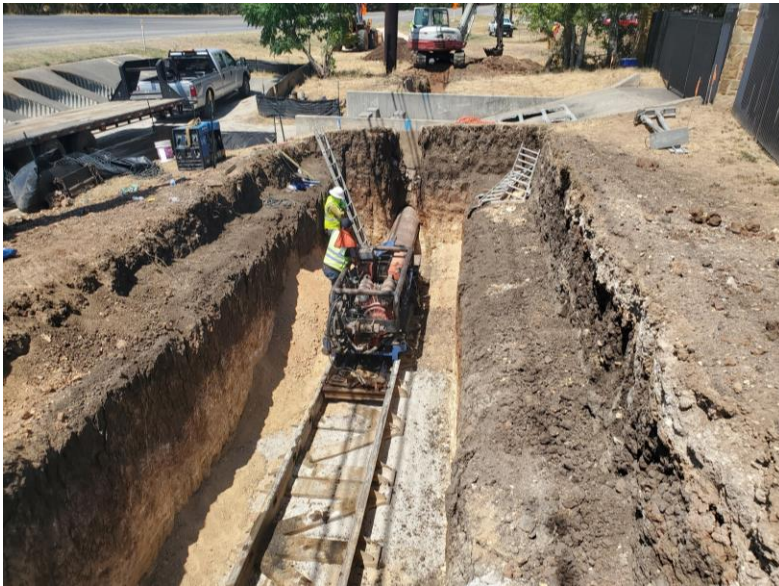
Bored 24-inch Steel Casing Under Arrowood Drainage Structure Approximately STA. 236+87
